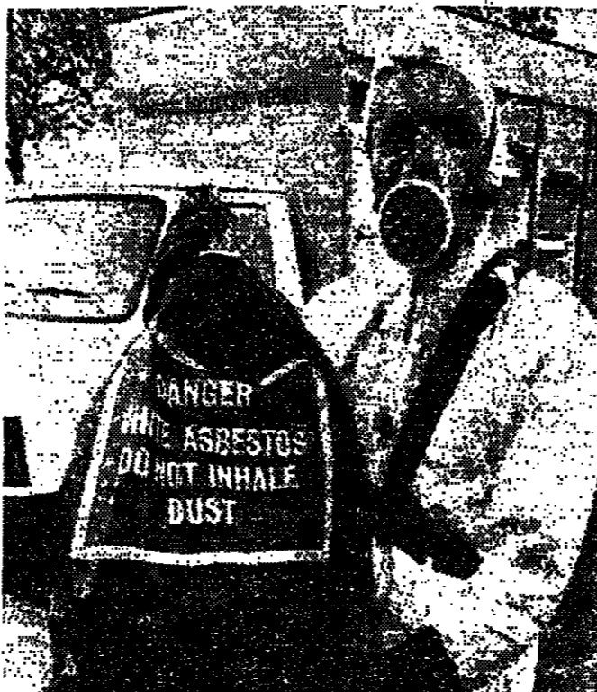
Asbestos danger: special equipment used by the GLC to clear contaminated sites. Asbestos is responsible for a mass of insurance claims adding to the strain on Lloyd's
